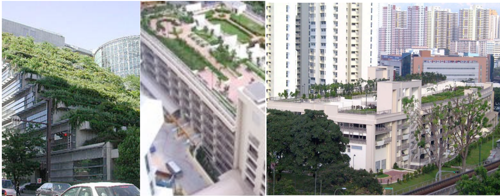
Parking Block Roof Garden, Queenstown, Singapore
